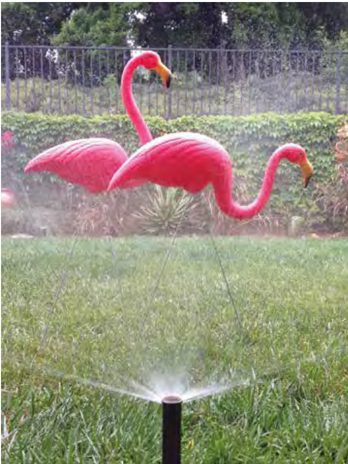
IMPROPER INSTALLATION – No flexibility
